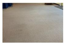
The carpeting in the vestibule and the office wing has reached the end of its useful life and needs to be replaced. It soils easily and cleaning can only do so much. It should be replaced with a long-lasting, high-traffic solution.
