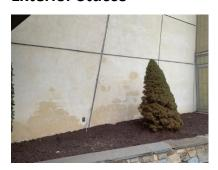
The exterior stucco on the building needs to be repaired and recoated. This is standard maintenance on the material.
