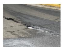
There are numerous potholes and cracks on the parking lot. It does not currently need to be milled and replaced, but the problem areas need to be patched and the entire surface resealed.
